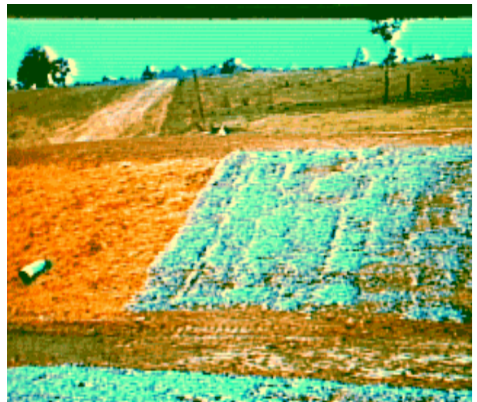
Mulching as a Best Management Practice to Reduce Soil Erosion and Infestation of Noxious Weeds Photograph provided by Libby Y. Field and Bernard A. Engel
